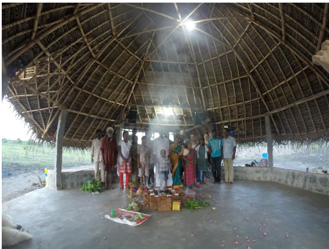
LIVING QUARTERS STRUCTURES: BAMBOO, TREE BRANCHES, WOODEN POSTS AND PALM FRONDS.
